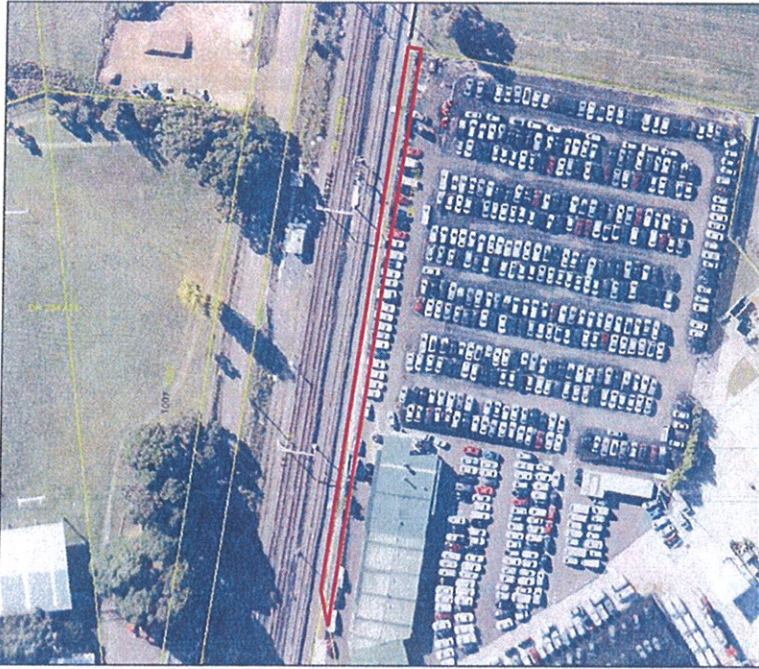
Figure 34: Aerial Photograph of Lot 10, DP 776165
